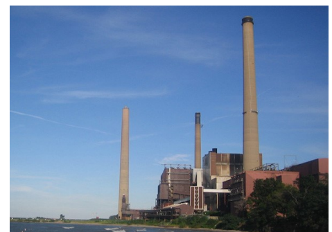
Avon Lake power plant
